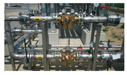
Dome to be isolated. This parallel arrangement gives 100 % up-time.
